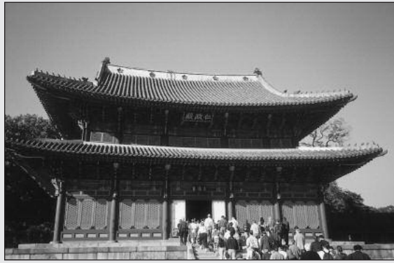
Old style building of the Changdok Palace of the "Chosen Dynasty."
